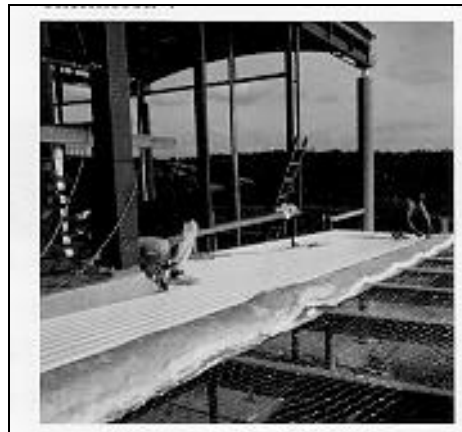
Flat Metal Deck Roof With Ceiling Lining
